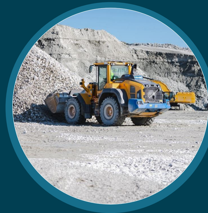
Excavated masses from pool pits...
