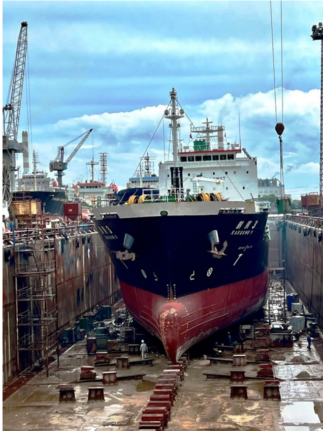
Traditional dry dock
