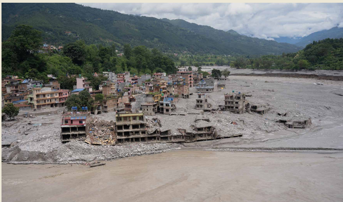
Houses damaged by the flood in Trishuli Bazaar, Nuwakot. Credit: Sharada Bashyal/Oxfam
