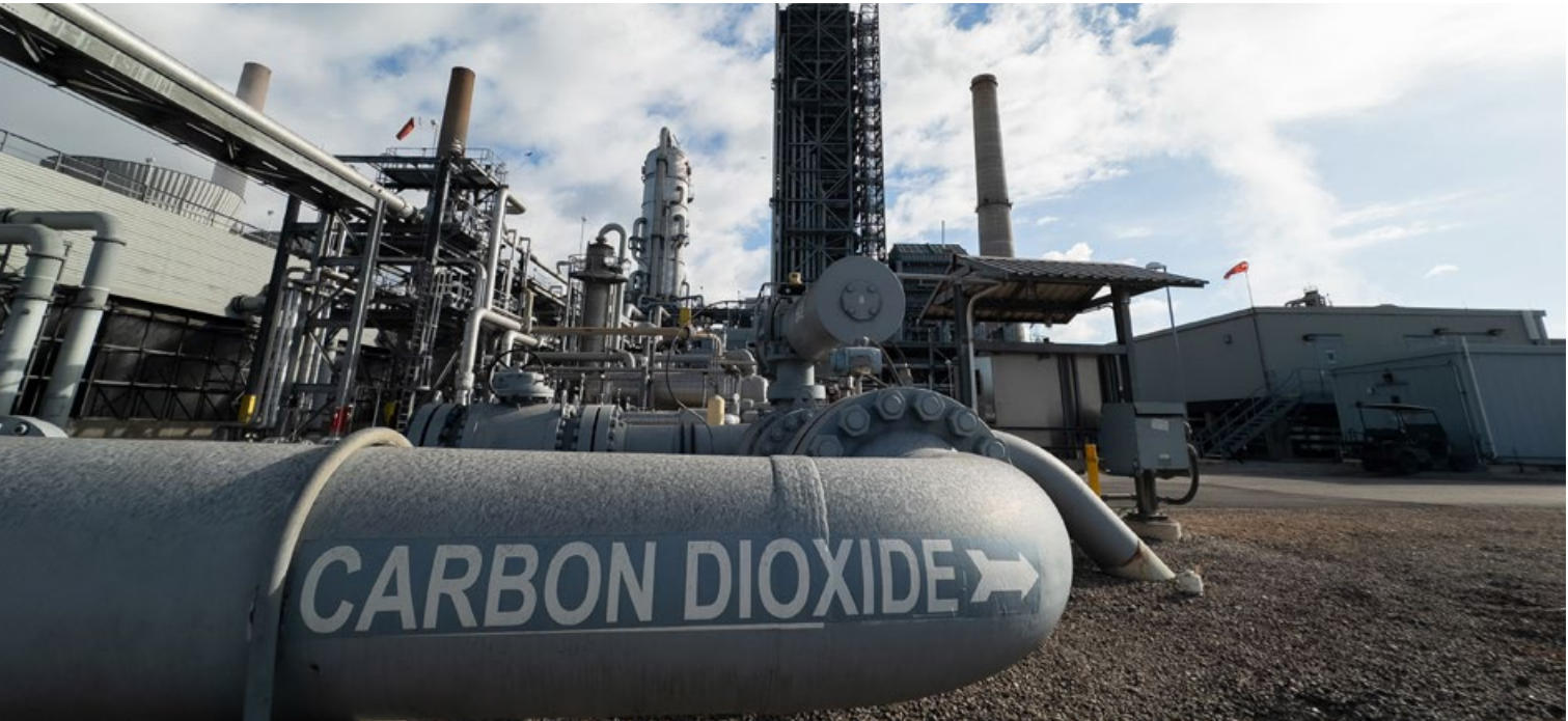
The Petra Nova facility that captures CO 2 from post-combustion flue gas at NRG’s W.A. Parish coal power plant in Texas, USA. Image courtesy of Petra Nova facility owner, ENEOS Xplora Inc.
