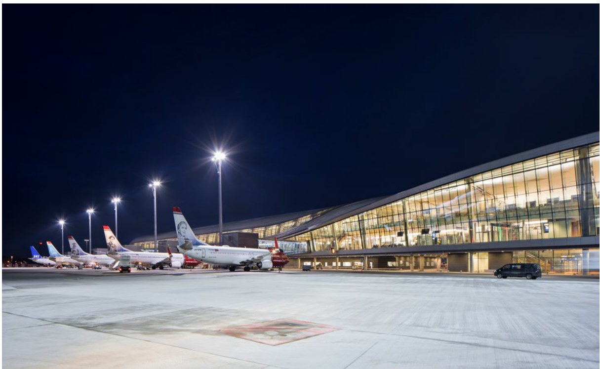
Figur 2.1: Oslo lufthavn. Kilde: Avinor - Nordic Office of Architecture - Ivan Broderly
